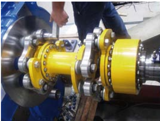
Ixilflex® during installation.
